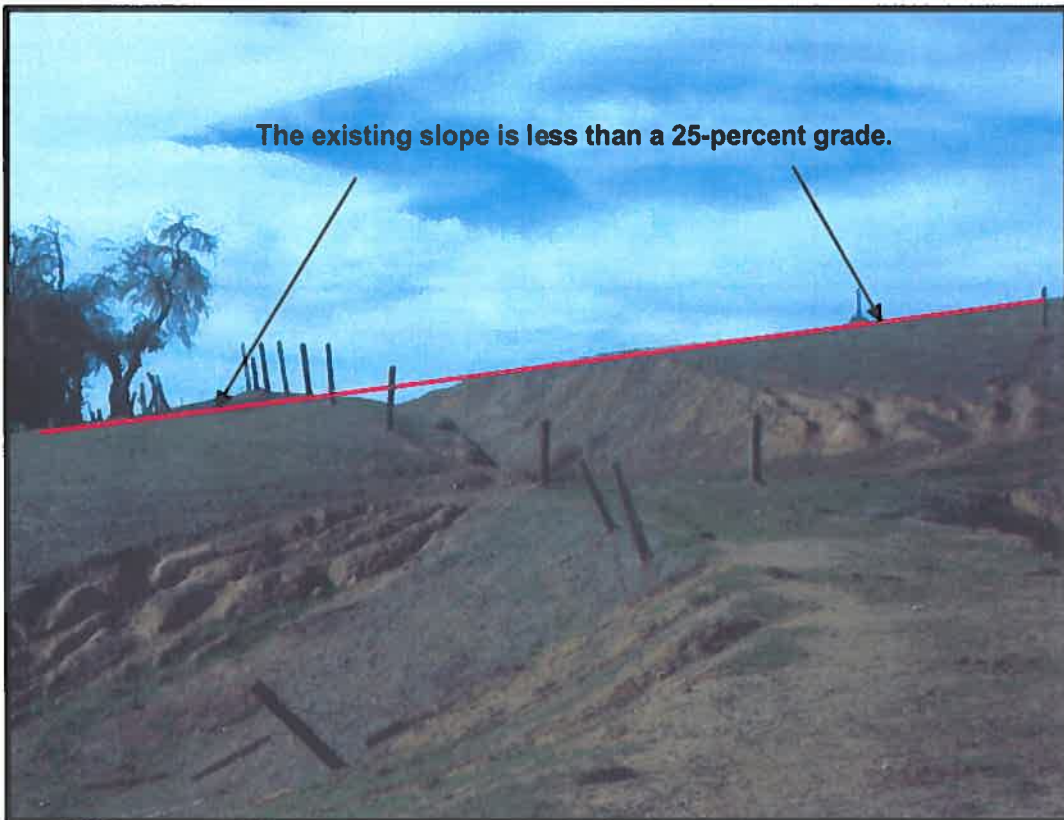
Figure 7: Looking Back at the Cut Slope in Figure 7.
